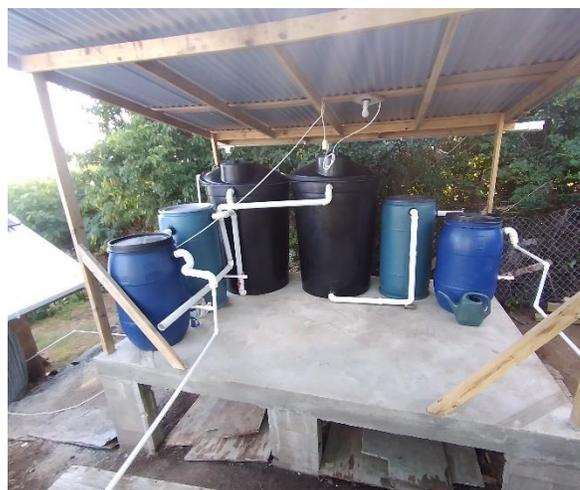
Completed platform area with roof that facilitates additional rainwater catchment for PMWIA’s aquaponics system. © PMWIA
