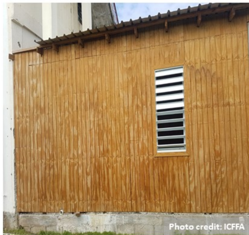
Image: Upgraded storage facility constructed by the ICFFA
