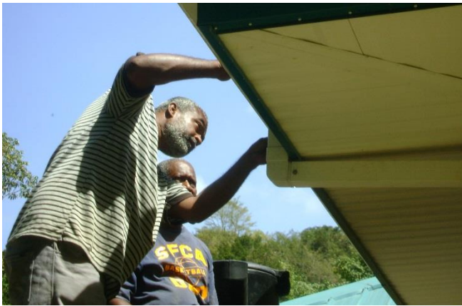
Caura residents install a rainwater harvesting system for their community centre
