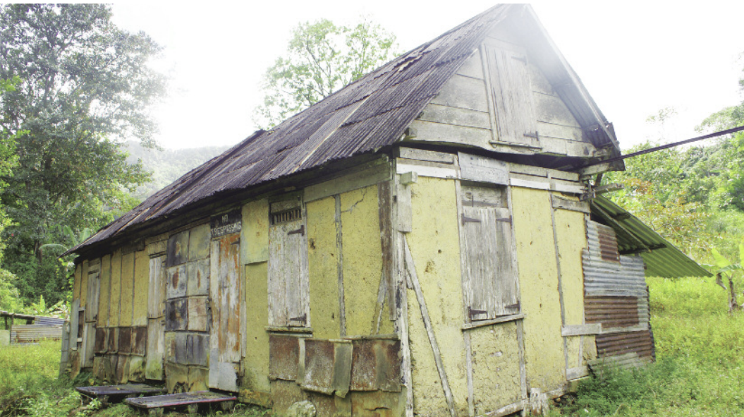
Figure 2: An old cocoa processing house in Trinidad
