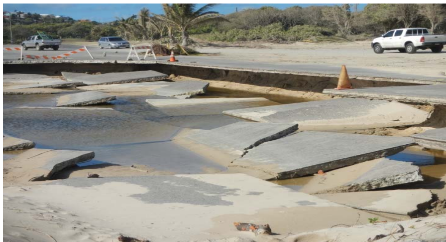
Figure 2: Destruction to the Vieux Fort Highway caused by seawater inundation. Without action more intense storms brought on by climate change will continue to cause costly damage to infrastructure. Photo credit: SLNT
